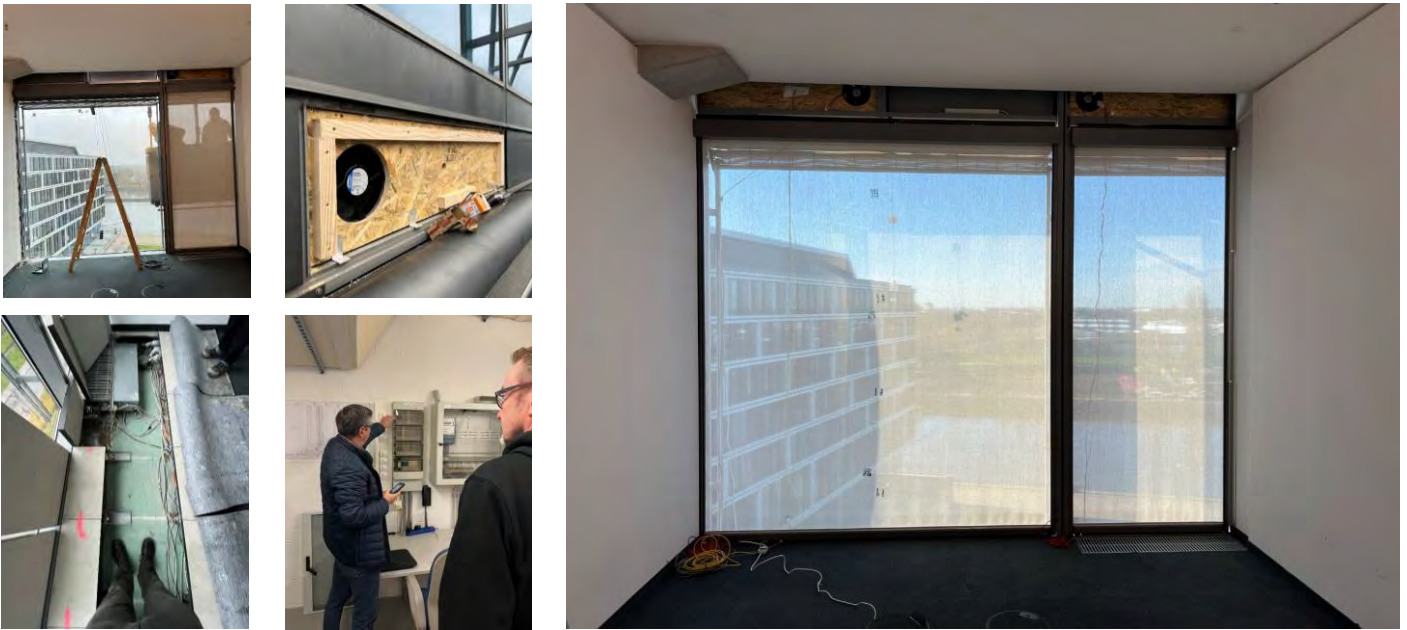
Transformation into a test façade
