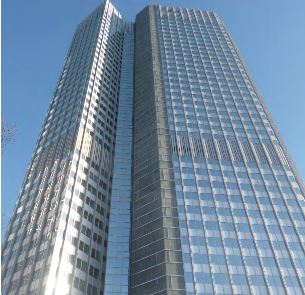
Facade elevation before refurbishment
