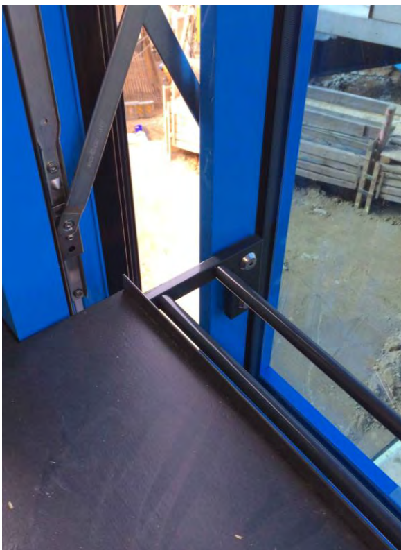
Mock-Up – Parallel-opening window with step protection
