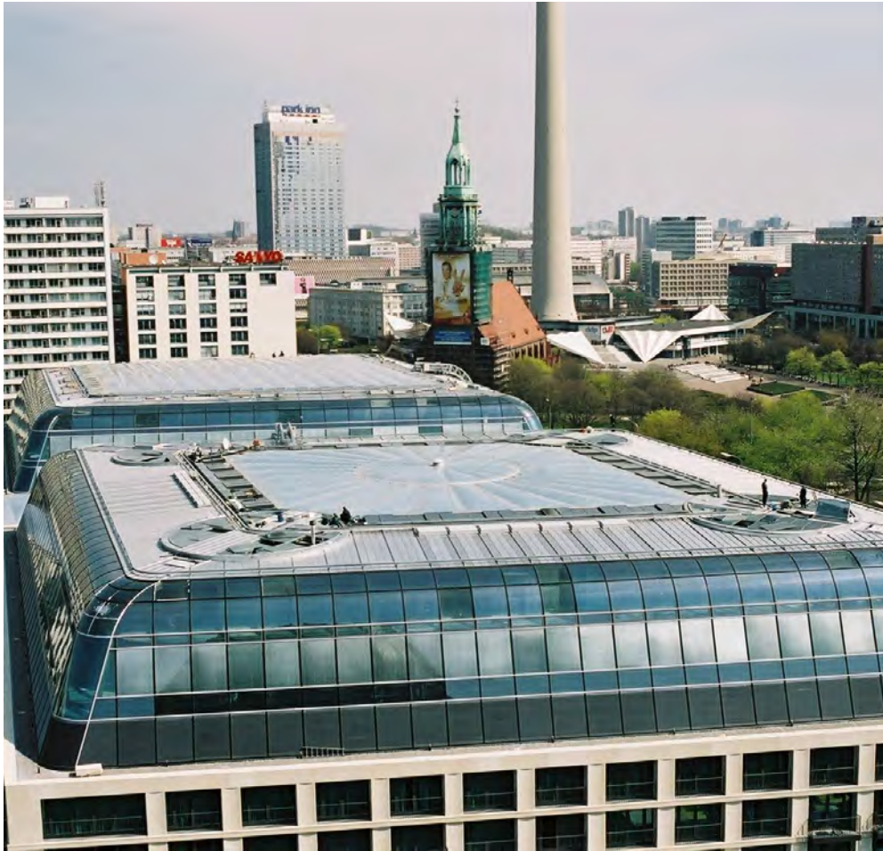
Aerial side perspective, inclined and bended glass roof glazing at the sides and foil roof in the centre
