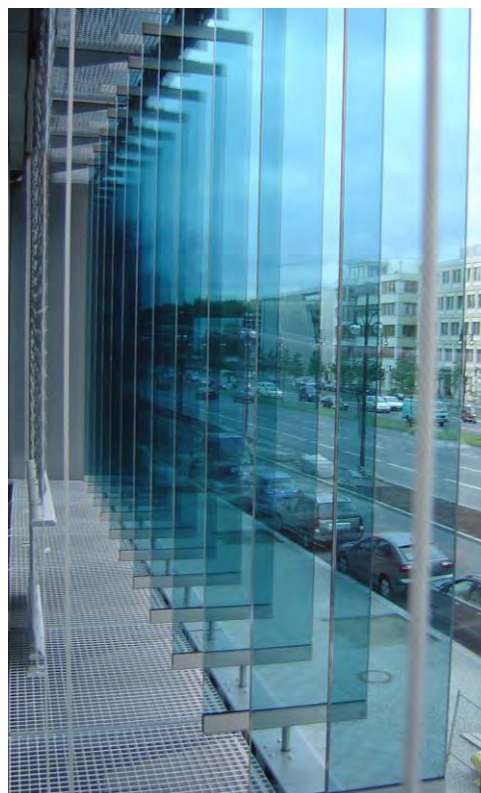
Unitized curtain wall with integrated walkway and rotatable vertical lamellas, external sunshade in open state
