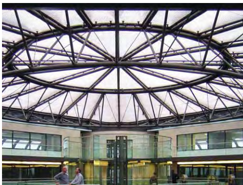
Foil roof structure as seen from below
