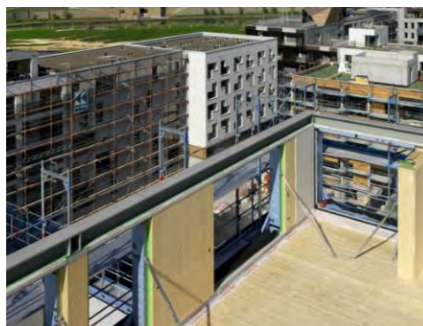
During construction progress
