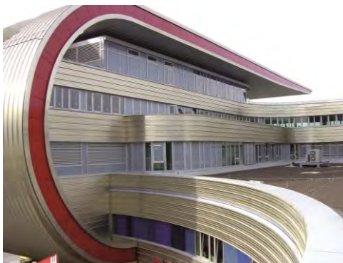
Curved aluminium standing seam profiles
