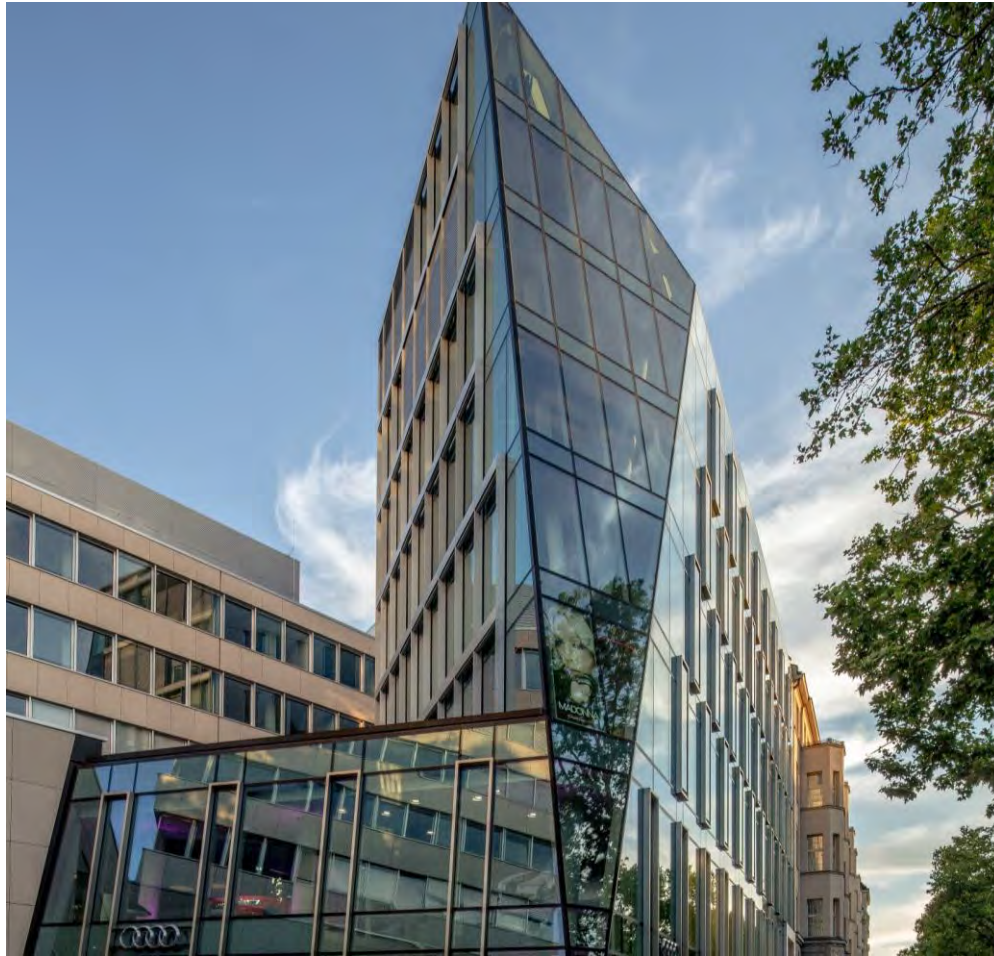
The extension building at Kudamm N°195, view from the Kurfürstendamm
