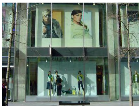
Stick system facade on the first levels
