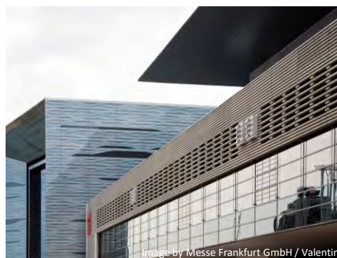
Facade elevation of exhibition hall 11 with precast reinforced concrete units
