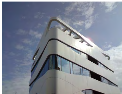
Facade elevation with a look at the building edge
