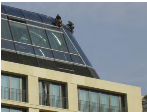
Inclined and bended roof glazing, window cleaners at work
