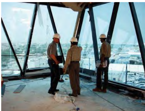
Site installation check
