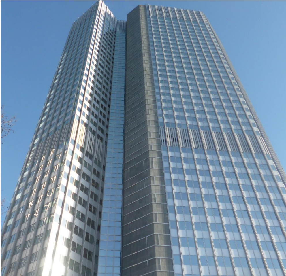
Facade elevation before refurbishment
