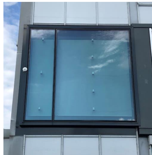
VERU test facade
