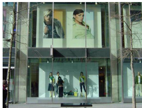
Stick system facade on the first levels
