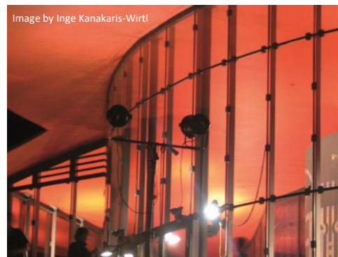
Facade elevation of point fixed glazing
