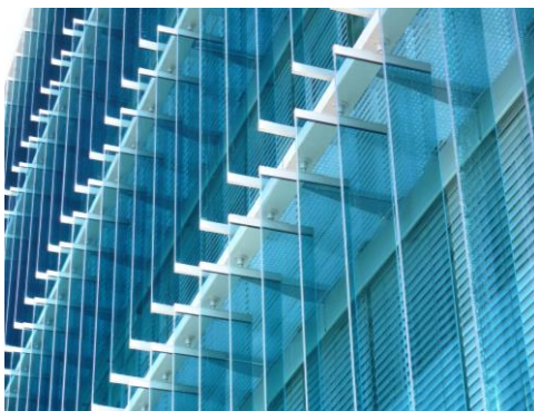
Controlled, vertical glass lamellas as-built
