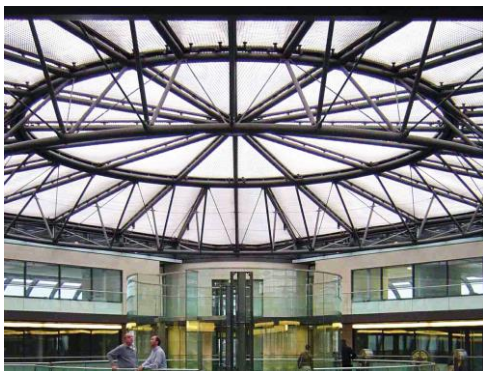
Foil roof structure as seen from below
