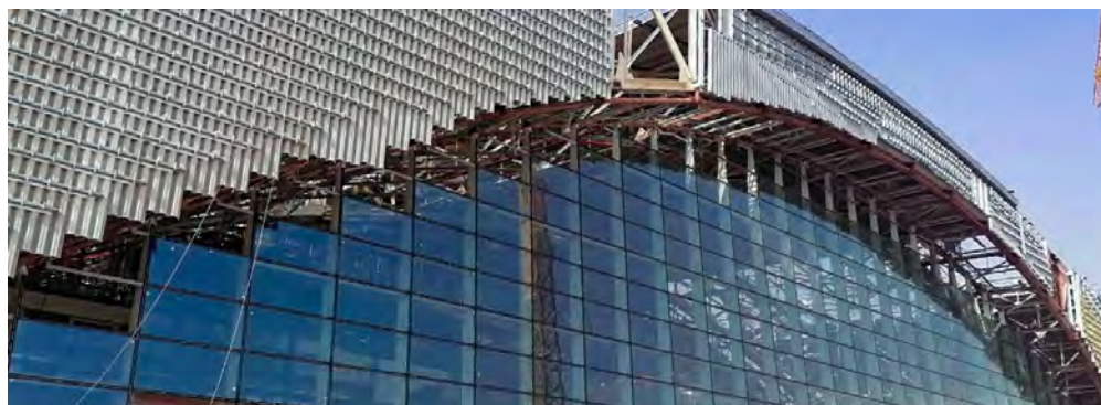
External facade during construction in progress
