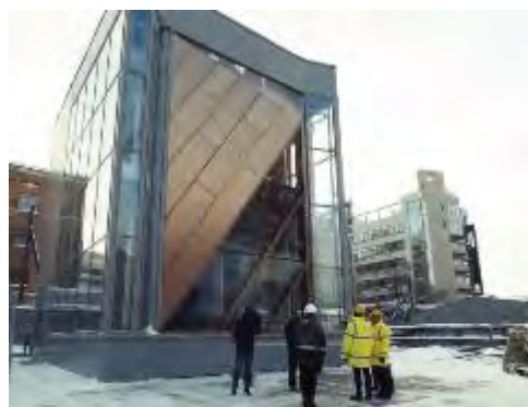
Mock-Up on site, January 2017
