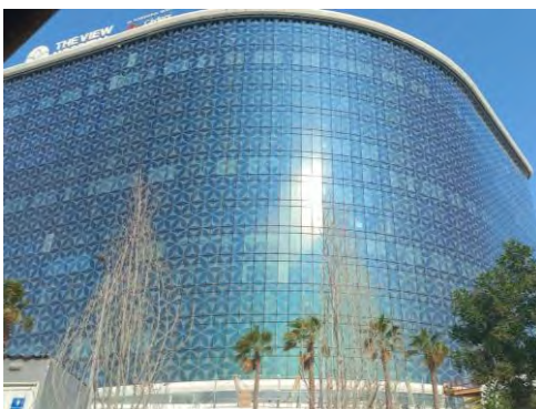
Under construction, almost finalized
