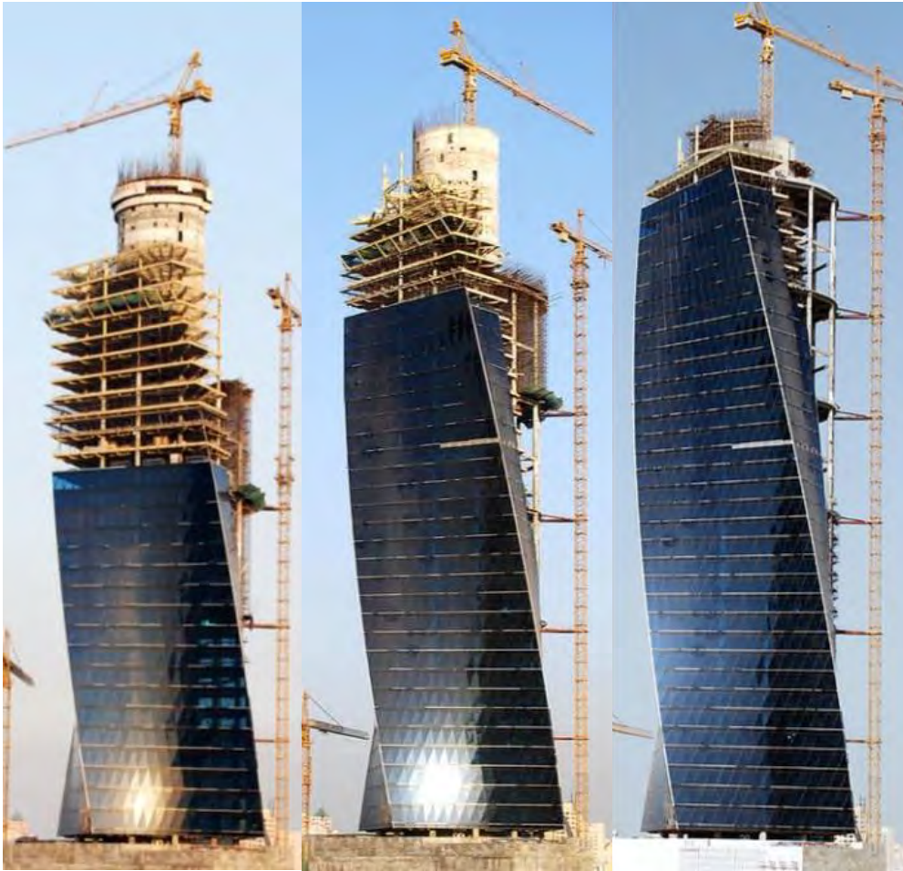
Progress of construction work
