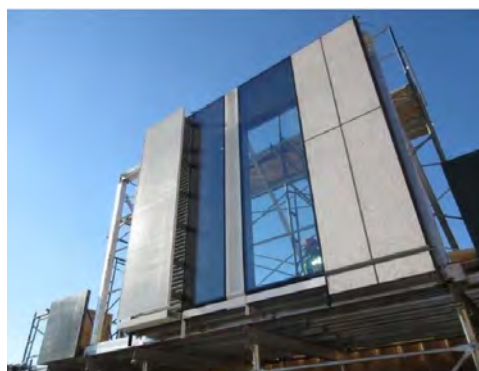
Visual Mock-Up in progress, February 2016
