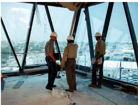
Site installation check
