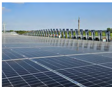
PV-roof and elevation of steel-substructure with PV elements
