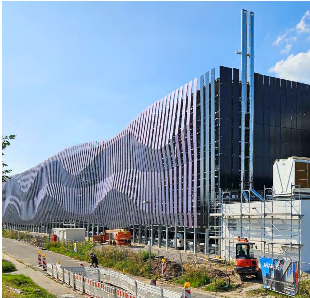
DHL-Campus, car park façade during construction progress, August 2023
