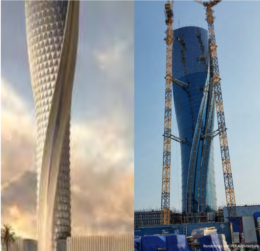
NPP Control Tower at twilight, rendering and the progress during construction
