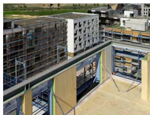
During construction progress
