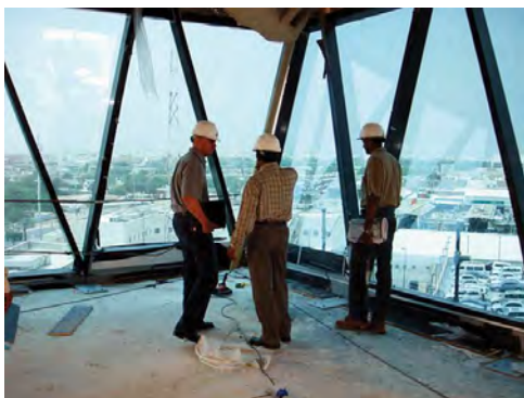
Site installation check
