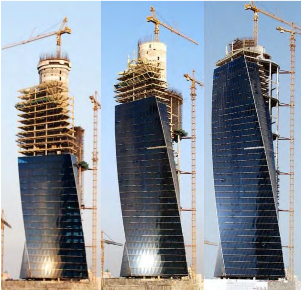
Progress of construction work
