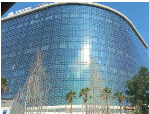
Under construction, almost finalized
