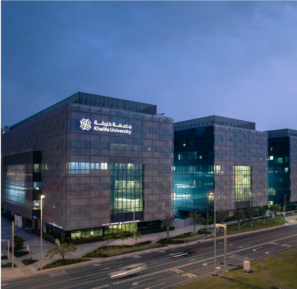
Khalifa University after completion
