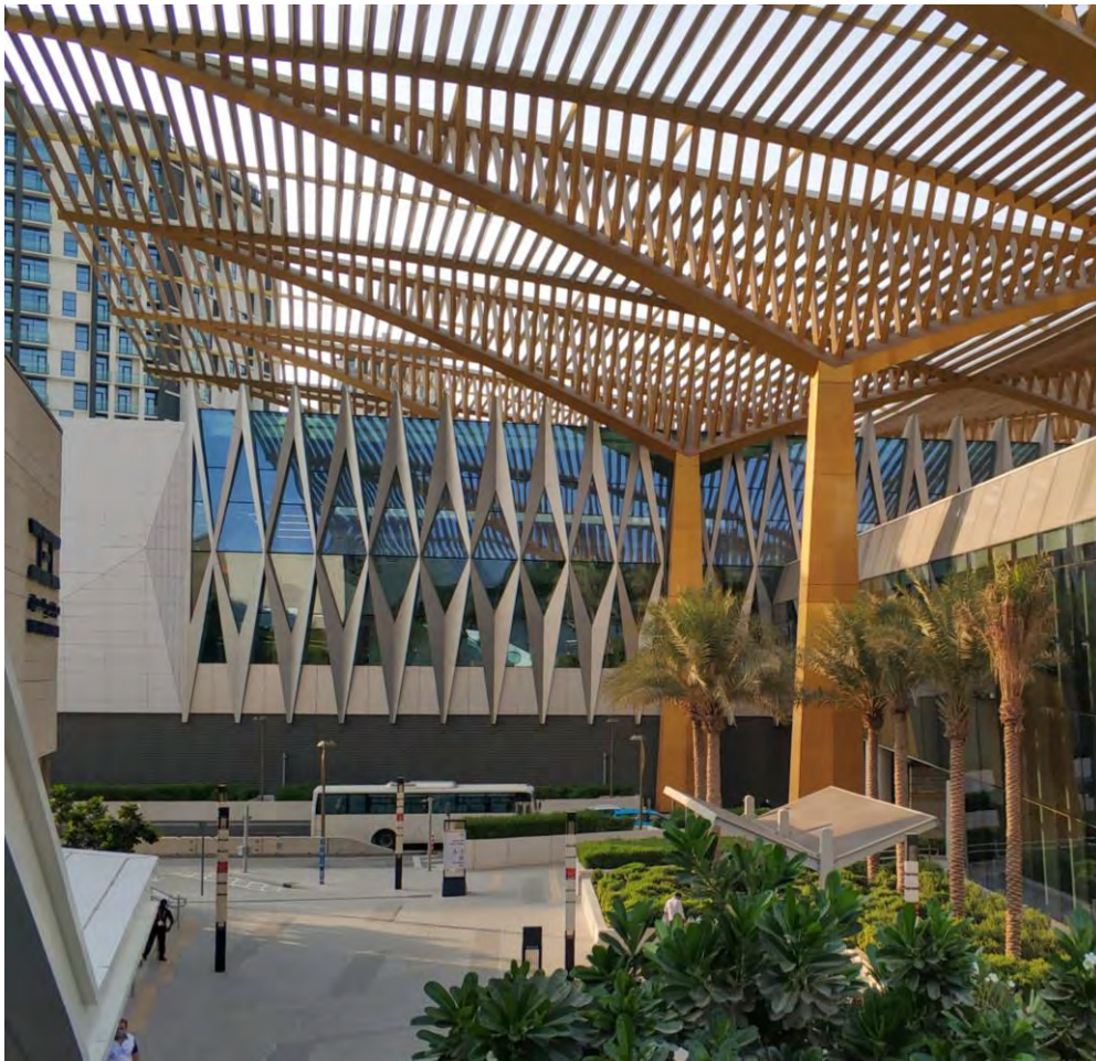
Expo 2020 Metro station on commissioning
